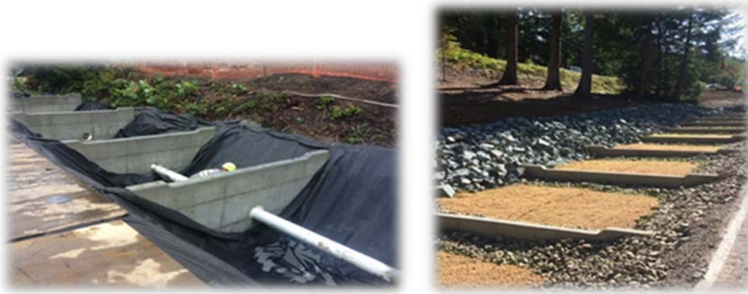
Figure 1. Lake Whatcom Cedar Hills-Euclid Stormwater Improvements
