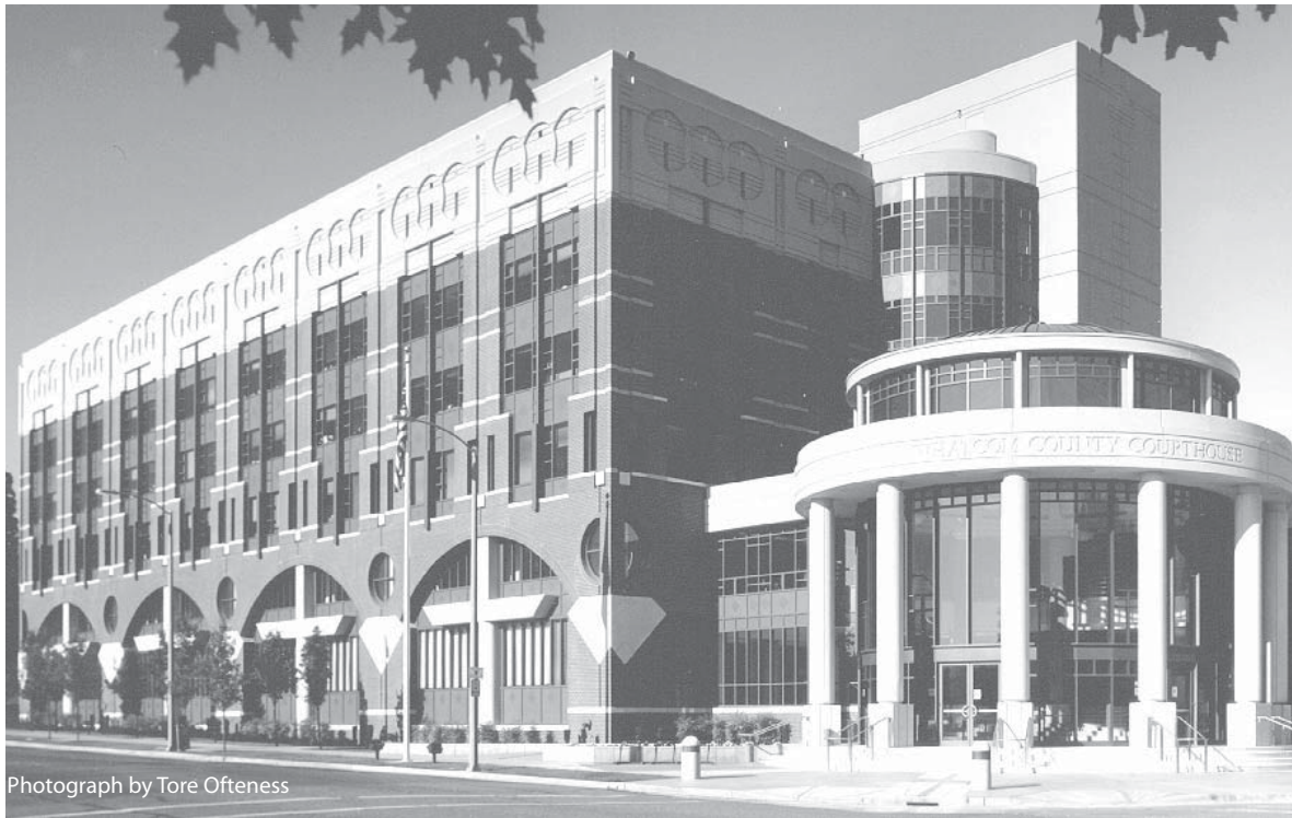
The Whatcom County Courthouse, 311 Grand Avenue, Bellingham, Washington.
