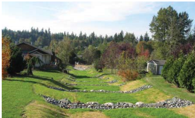
Silver Beach Creek Improvements – Brownsville Drive to E. 16th Place
