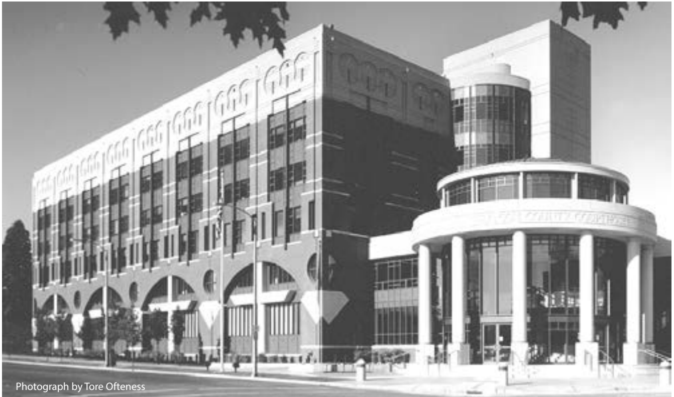
The Whatcom County Courthouse, 311 Grand Avenue, Bellingham, Washington.
