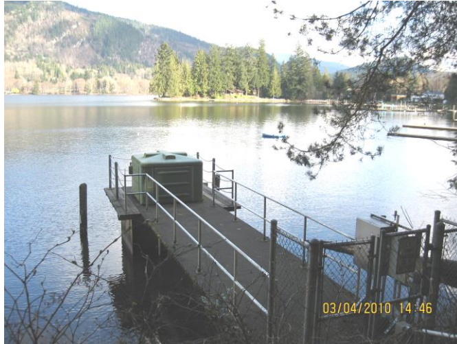
Photo 4-1. Sewer Pump Station Adjacent to the Lake
