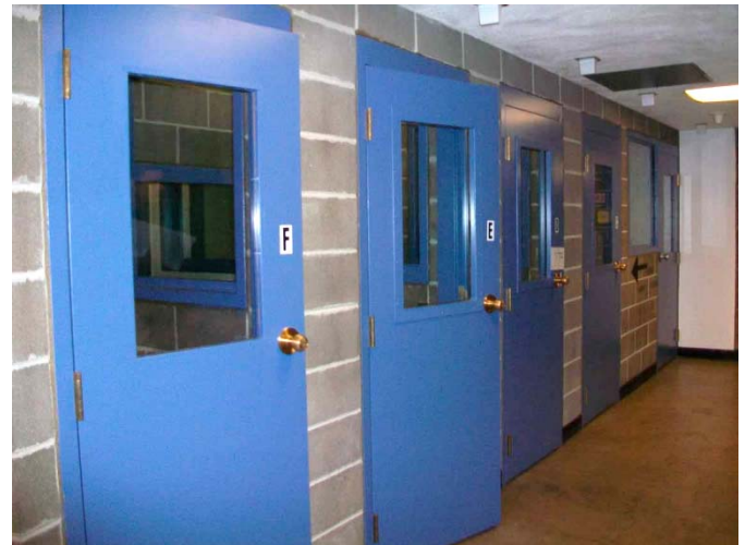
Figure 9.13: Looking towards inmate visitation doors
