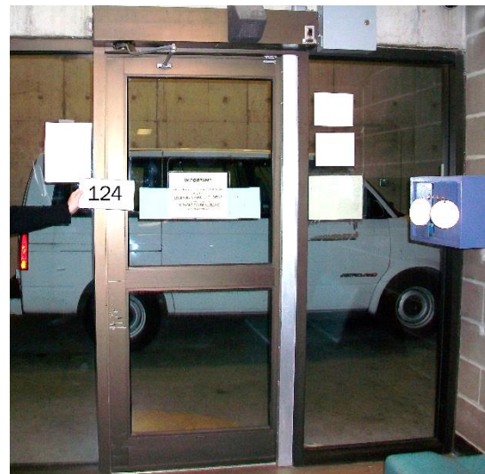
Figure 9.08: Door 124-Reception Side
