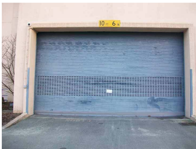
Figure 9.17: Standard condition of coiling doors
