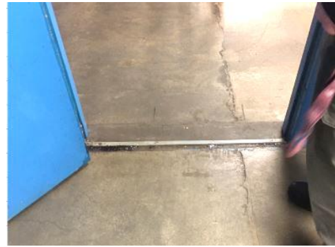
Figure 10.12: Metal Strip at Threshold
