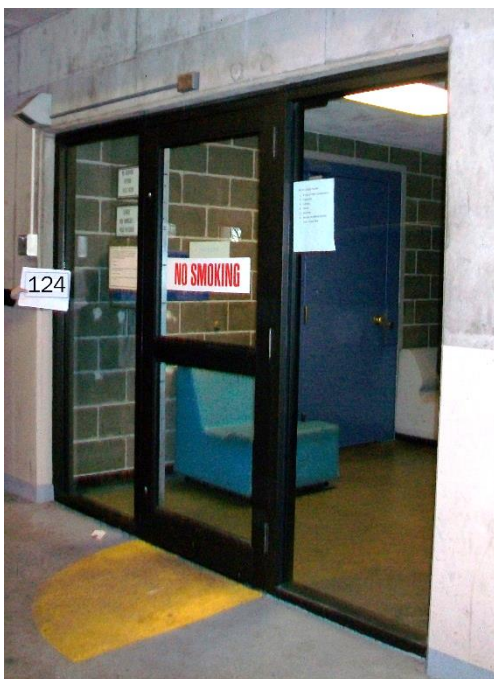
Figure 9.07: Door 124 -Sally port side
