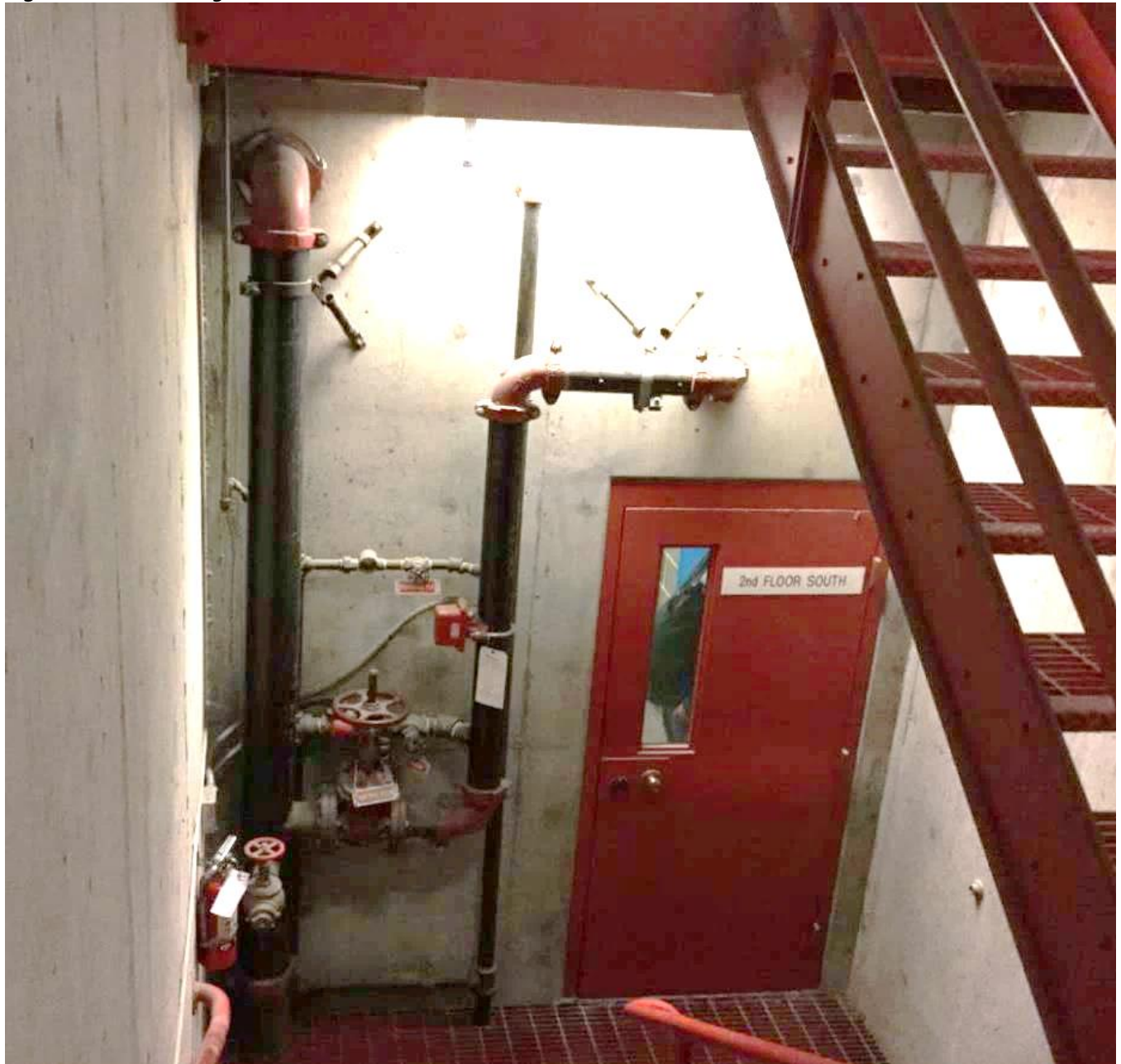
Figure 3/6.12: Bracing in stairwells.
