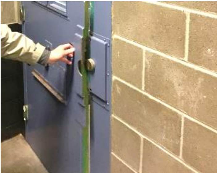
Figure 10.10: Recessed Hand Pull / Steel Cover Plate
